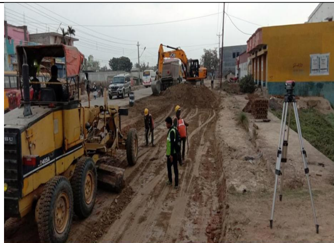
1st By-Pass, Preparation of Sub Grade and Sub-Base Work, Birgunj
